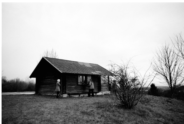
Figure 4. Log Cabin exterior, rear perspective.
