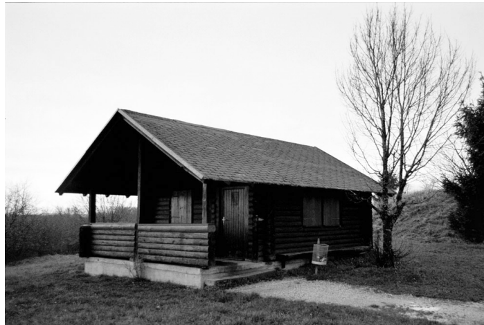
Figure 3. Log Cabin exterior.
